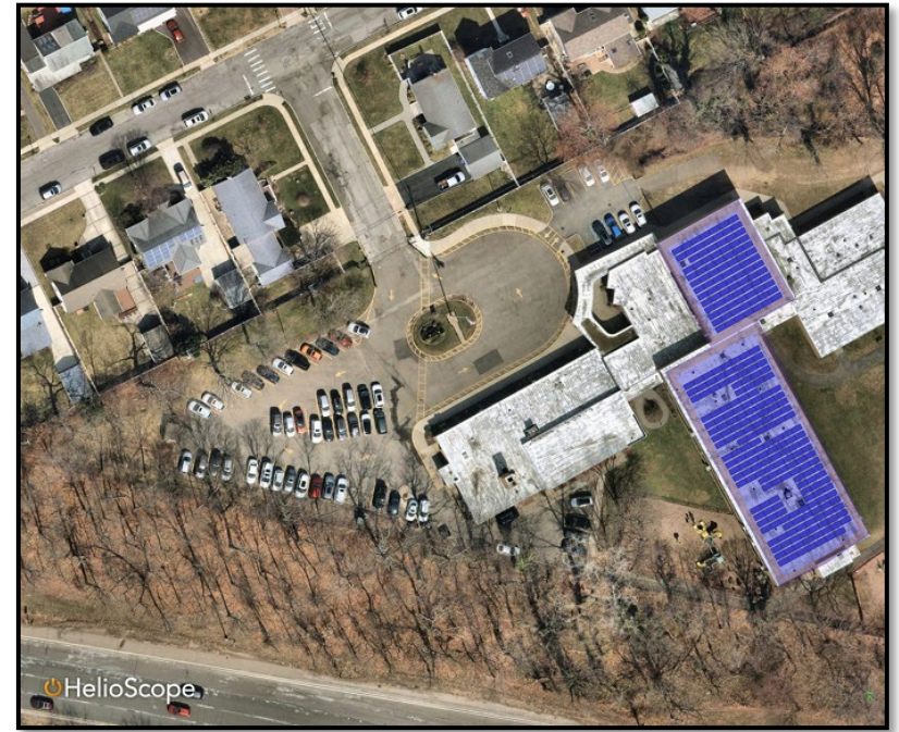
Lee Road Elementary School
